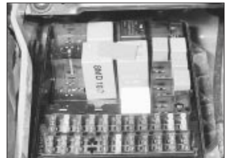
3.3b Fusebox cover removed to expose fuses and relays (1.8 CVH model shown)
