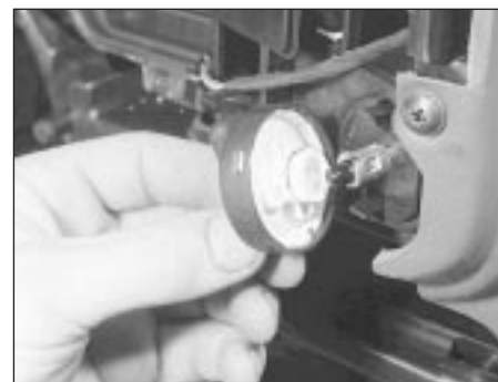
6.21 Pull off the switch knob to expose the bulb
