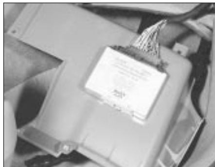
27.30 The bulb failure module secured to the under-dash trim
