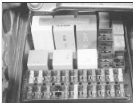
16.2 Main fuse/relay box under the bonnet
